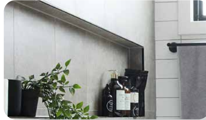
Shower Niche in Bathroom and Ensuite
