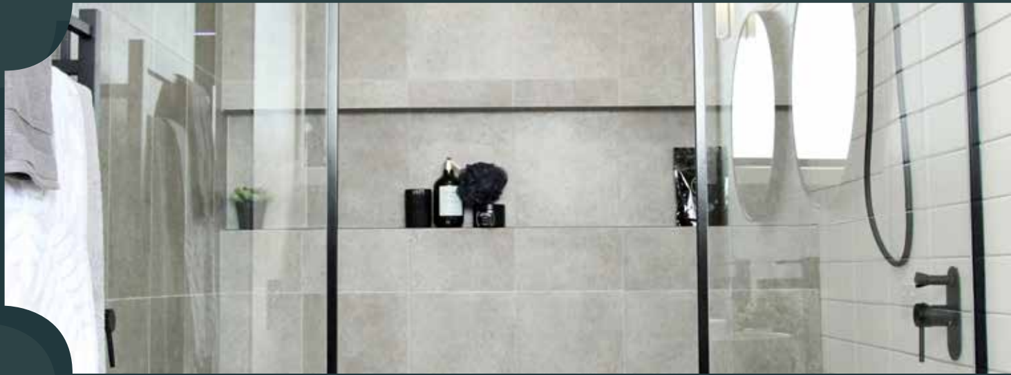
Full height tiling in Bathroom and Ensuite
